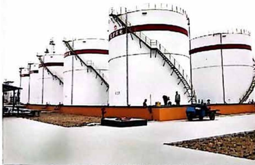
LIAONING YIFANG PETROCHEMICAL CO. LTD. VERTICAL STORAGE TANK PROJECT
